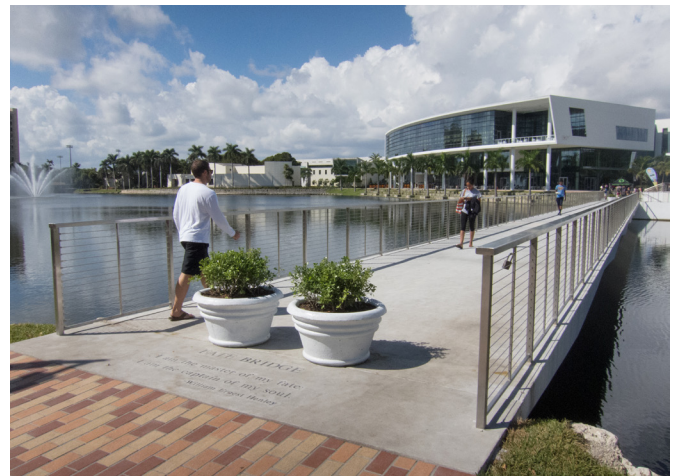
Fate Pedestrian Bridge
