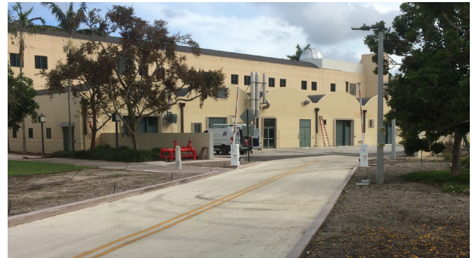
Controlled Access Service Road behind Physics
