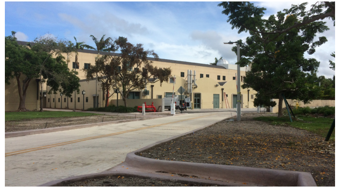
Controlled Access Service Road behind Physics Building
